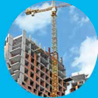
INSTALLATION AND DELIVERY
